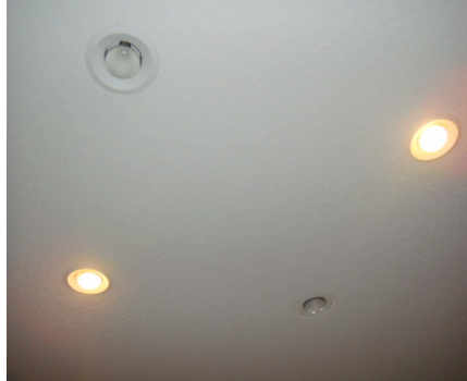
Burnt out light bulbs
