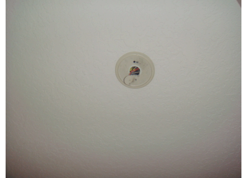
Missing smoke detector
